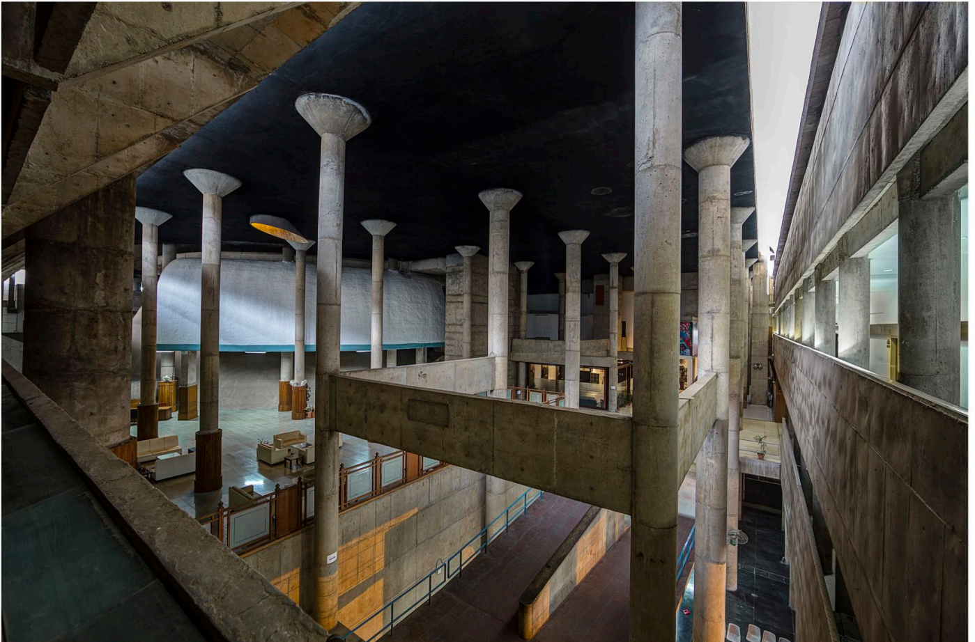
Chandigarh, Palace of Assembly (Vidhan Sabha) (1951-64). Interior View with Columns and the Ramp, 2014 Canson Platine Fibrerag Variable sizes
